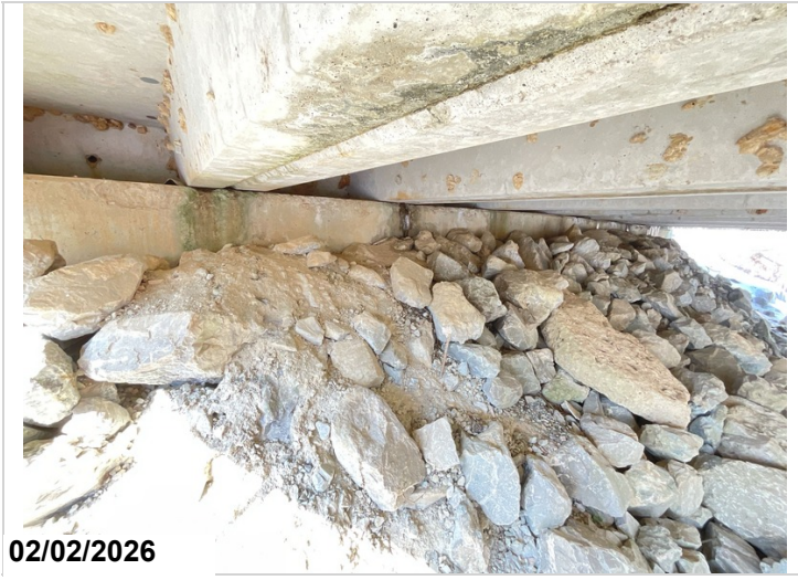
Minor chips/spalls under units
